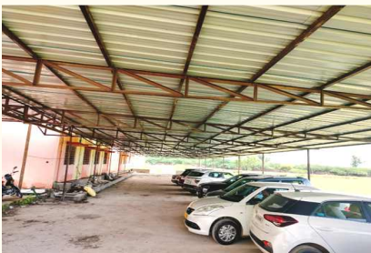
Construction of Parking Shed at ARS Ummedganj, Kota
