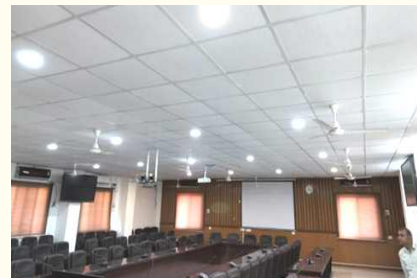
SITC of Split AC at ATMQIC Building at AU, Kota
