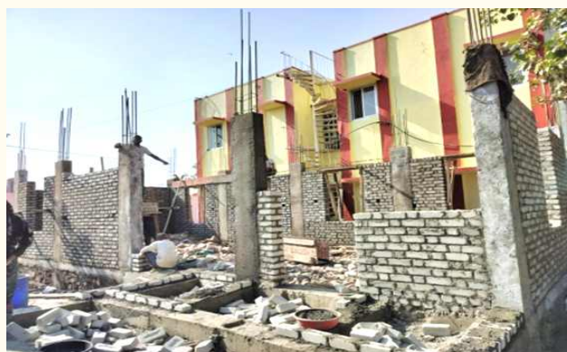
Construction of Skill Development Hostel for trainee at AU, Kota
